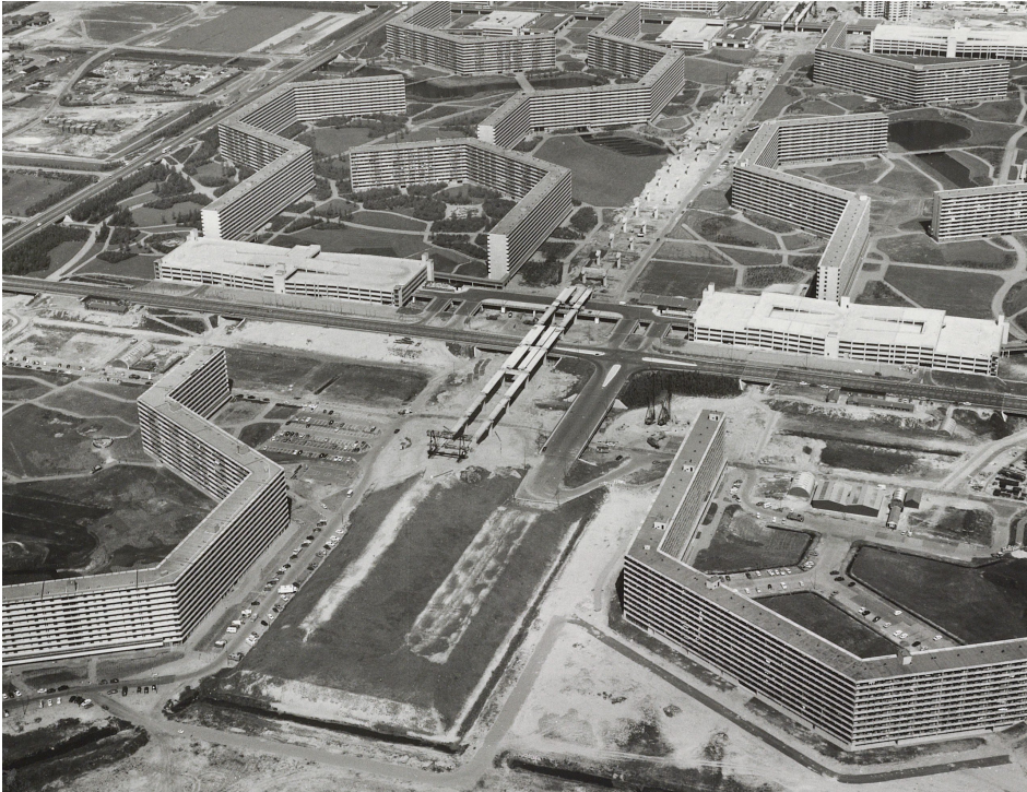
Fig. 2: The Bijlmer under construction in the early 1970s.
