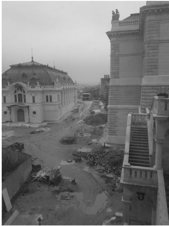
Image 3: Finishing the full reconstruction of the “Wrangler Court” ( Csikós udvar ) with the Riding Hall (left) in December 2019. The Riding Hall was built in 1899-1902, partially destroyed during World War II, and completely demolished in 1950. Its reopening as a 1500 sqm event hall is due in 2021.
